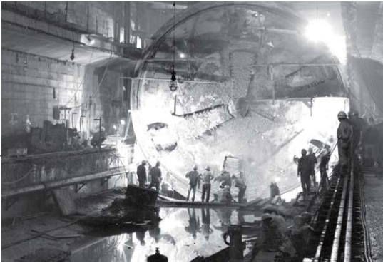
Work underway on constructing the Namba underground line (1969)
