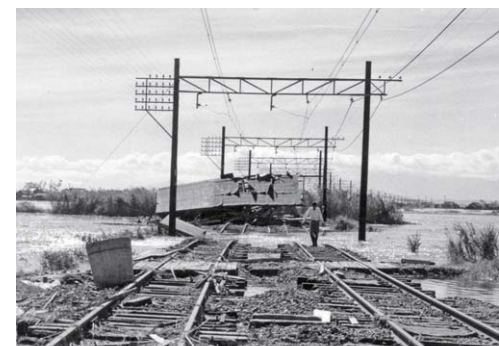
The Nagoya Line Suffered Damage in Typhoon Vera (1959)
