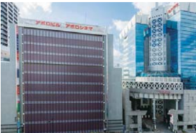
Apollo Building and Lucias Building
