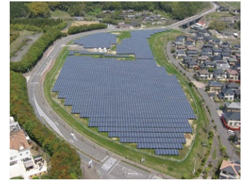
Kintetsu Oita Takae Solar Power Plant (Oita City, Oita Prefecture)
