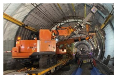
Anti-seismic reinforcement work on a shield tunnel on the Namba Line
