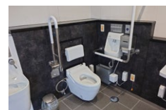
Accessible toilet installed in FY2024 at Miminashi Station
