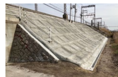
Embankment strengthening work (between Kintetsu-Koriyama and Tsutsui stations)
