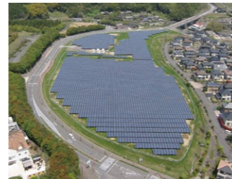
Kintetsu Oita Takae Solar Power Plant (Oita City, Oita Prefecture)
