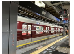
Platform edge gates with cables (Platform 2 at Tsuruhashi Station)
