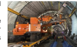
Anti-seismic reinforcement work on a shield tunnel on the Namba Line
