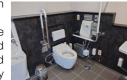
Accessible toilet installed in FY2024 at Mirinashi Station
