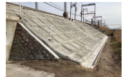
Embankment strengthening work (between Kintetsu-Koriyama and Tsutsui stations)
