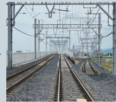
After work was completed
