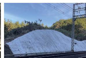
Embankment strengthening work (Osaka Line)
