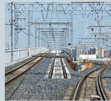
Before work to elevate the outbound line
