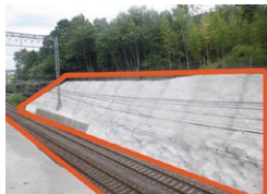
Line embankment strengthening
