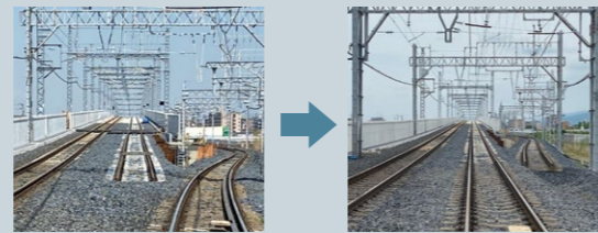
Before work to elevate the outbound line
