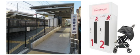
Ramps at Hozenji Station Sharing services
