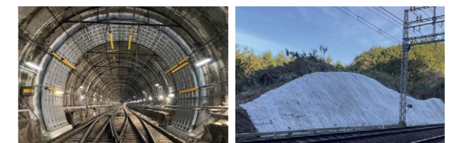
Anti-seismic reinforcement work on a shield tunnel on the Namba Line
