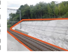
Line embankment strengthening
