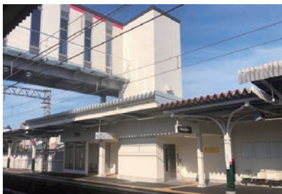
Accessibility (installing elevators)
