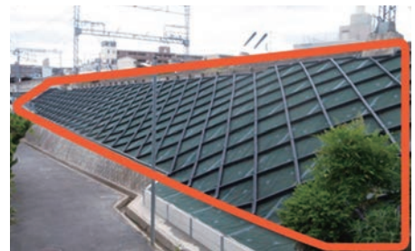
Embankment strengthening
