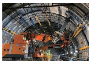
Anti-seismic reinforcement work on Namba Tunnel
